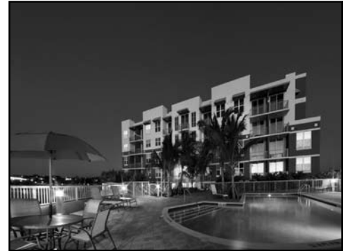
Progresso Point's pool deck and amenities on top of the three-story parking garage
