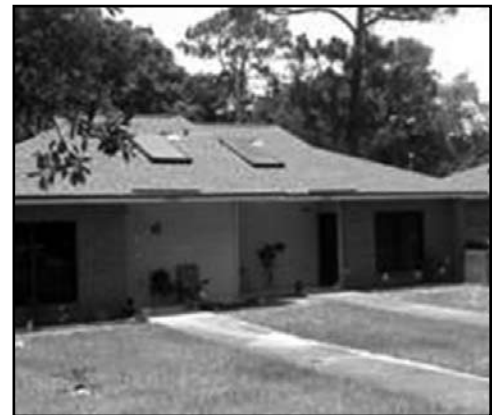
Solar panels are saving energy and money for Pensacola AHC residents.
