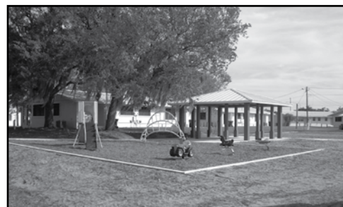
The new tot lot at Lakeside Park is ready for children to come and play.
