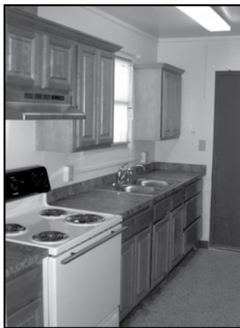
New cabinets await residents in this renovated kitchen at Lakeside Park.
